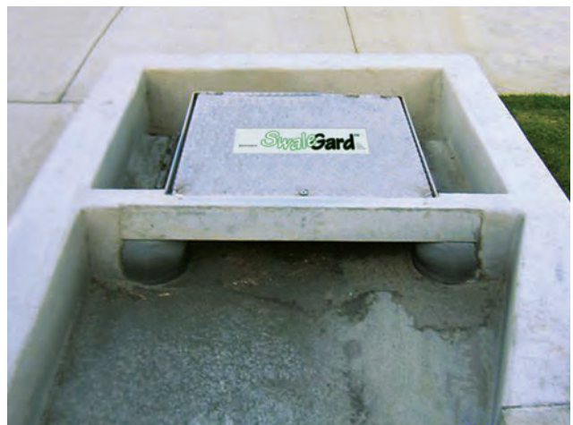
Installation in parkway culvert
