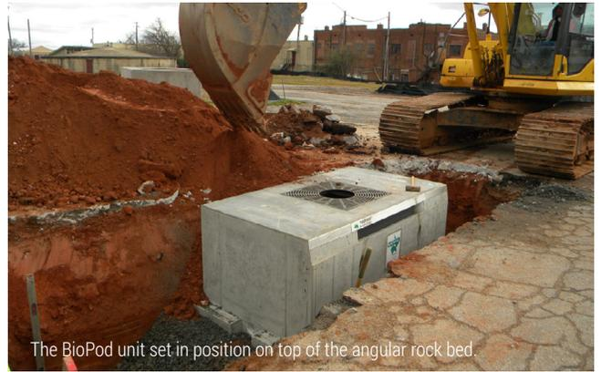
The BioPod unit set in position on top of the angular rock bed.
