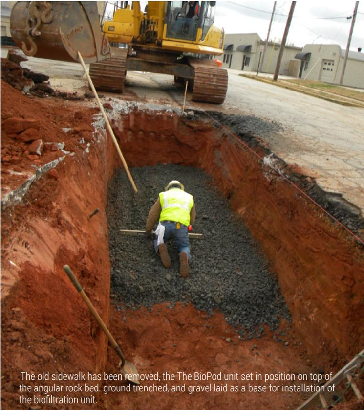
The old sidewalk has been removed, the BioPod unit set in position on top of the angular rock bed, ground trenched, and gravel laid as a base for installation of the biofiltration unit.
